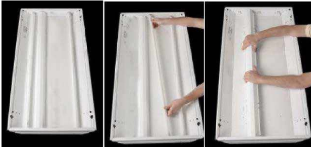
a) Troffer and lamps b) Remove tube lamps c) Remove ballast cover (lens removed)
